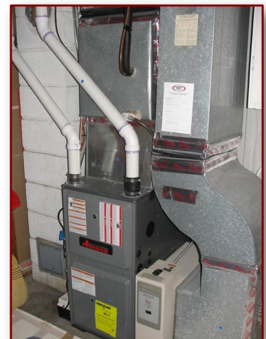
Their new, more efficient propane furnace.
